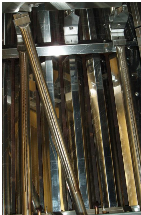
MAIN BURNER REMOVAL. PHOTOGRAPH 32.
