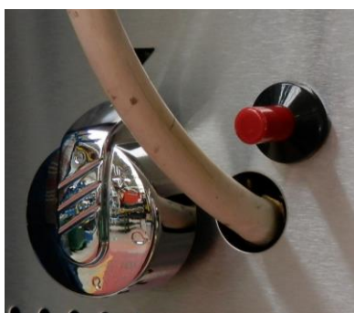
PHOTOGRAPH 21. GAS TEST NIPPLE.
