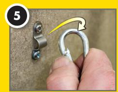
The restrainer wire can now be disconnected to allow free movement of the appliance.
